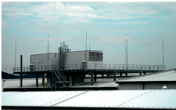
Insulated mast for elevated air terminals with high voltage cables
