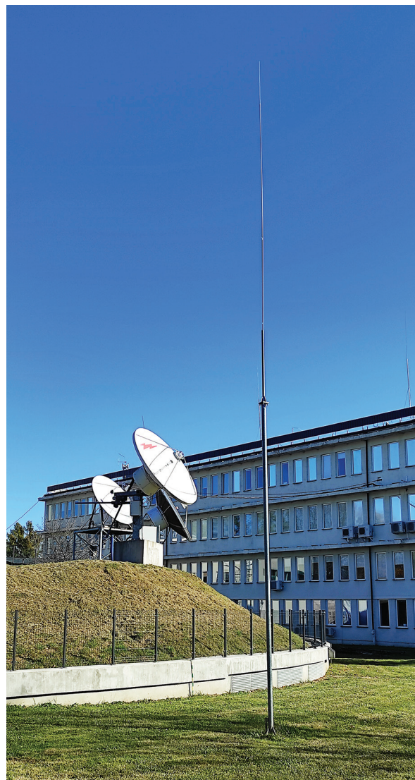
Mast on foundation H=13500mm AH35061
