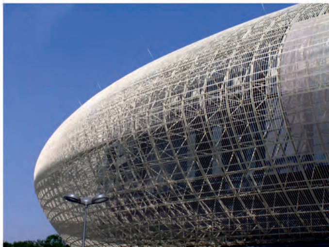
Insulated masts fixed to the structure of a sports hall to protect a LED screen.
