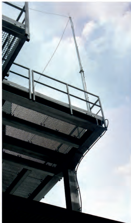
Insulated mast for elevated air terminals with high voltage cables
