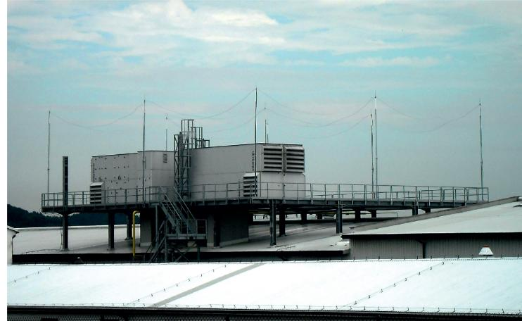
**Insulated mast for elevated air terminals with high voltage cables**
