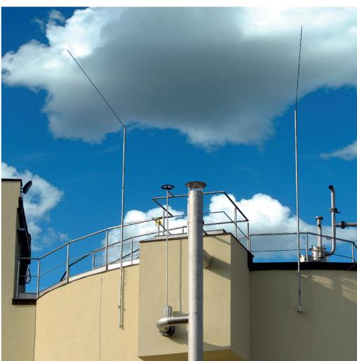
Bent masts to increase the protection angle of tank explosion zone..
